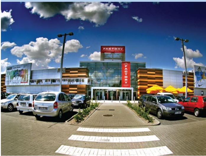
FACTORY OUTLET CENTER, POZNAŃ
