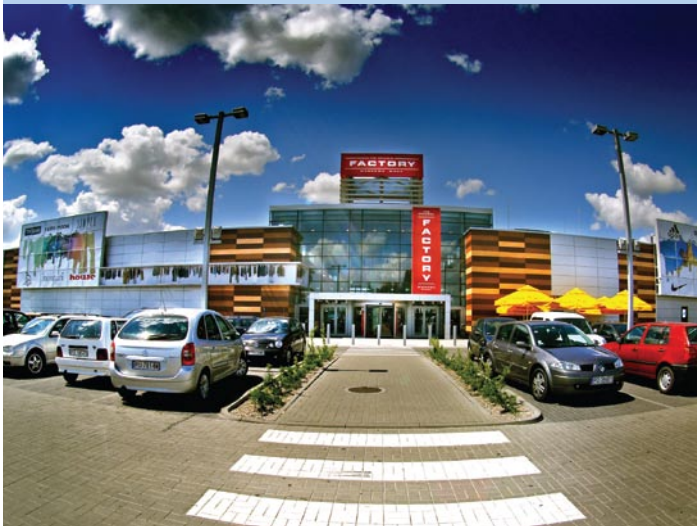
FACTORY OUTLET CENTER, POZNAŃ
